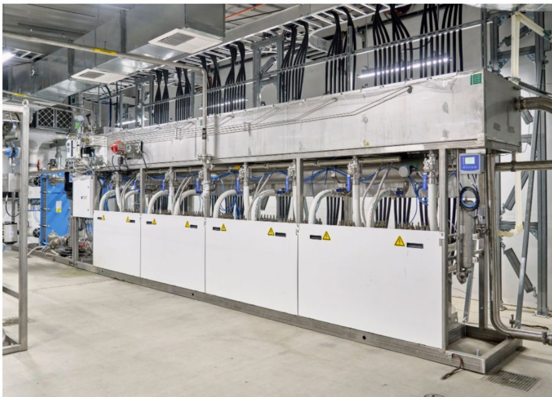
SunLine Transit has invested in equipment that can split water into oxygen and hydrogen atoms. Philip Cheung for The New York Times
